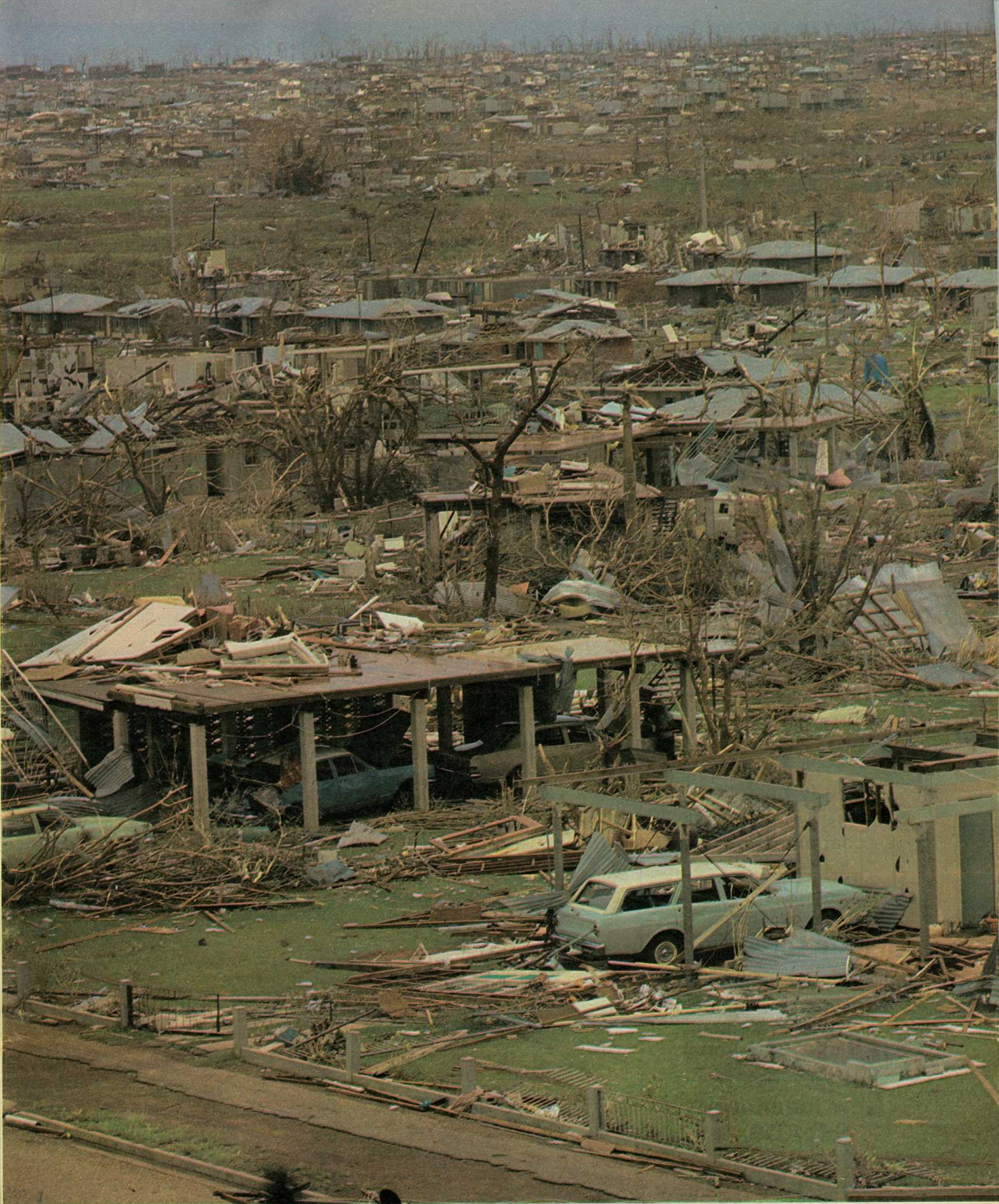
DISASTER AREA: Shattered homes in suburban Nightcliff, one of Darwin's worst affected districts. This picture was taken from the top of a still-standing apartment building.
