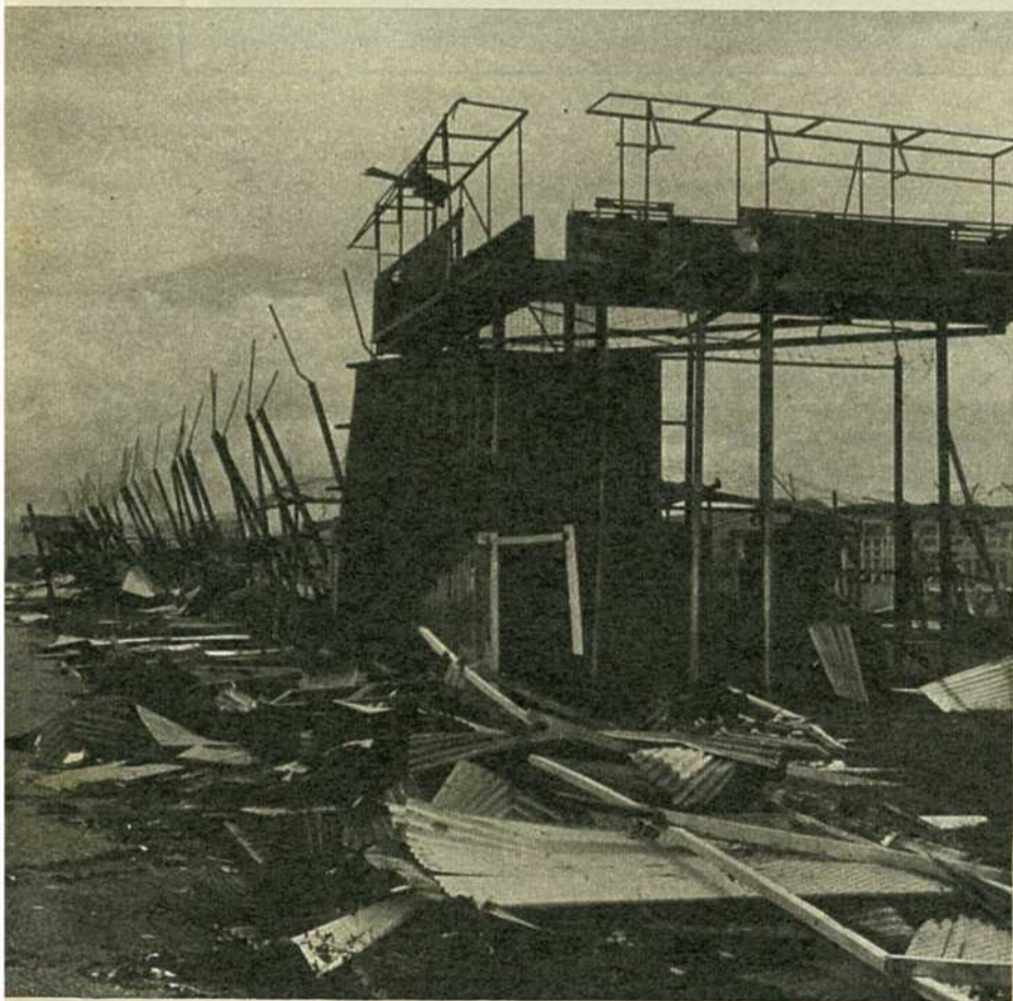
ABOVE: At Fannie Bay jail the force of the storm twisted and brought down steel fencing and partially destroyed one of the watch towers normally manned by guards.
