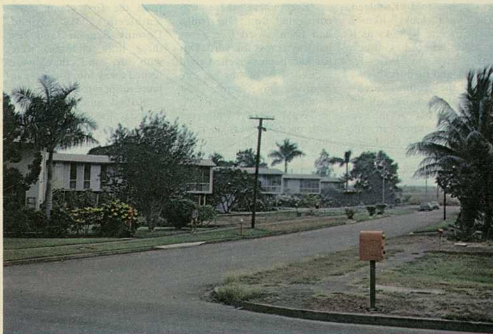
ABOVE: Darwin homes before Tracy hit. Experts are thinking about new building designs for Darwin so that it will cope more effectively with cyclones.
