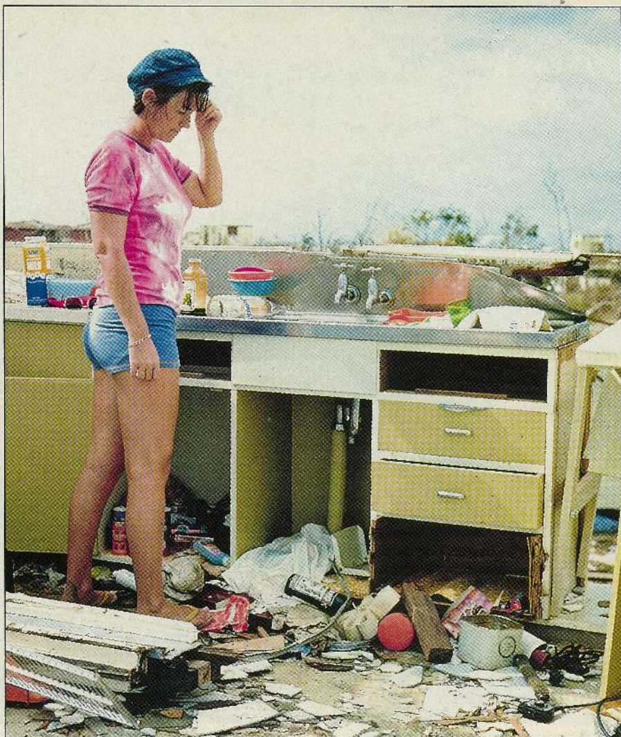
Darwin, Christmas morning, 1974: Muriel O'Connell sifts through the wreckage of the home of friends. Houses disintegrated under Cyclone Tracy's awesome force.
