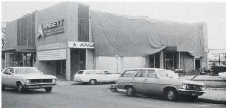
The office in Mitchell St., Darwin—not badly damaged when compared with many others.
